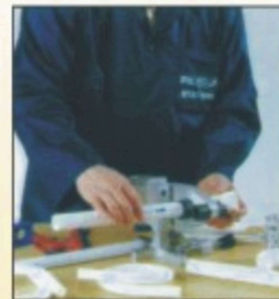
PIPE AND FITTINGS ARE HEATED...
